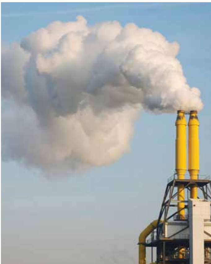
CDM Incinerators lack pollution control.
